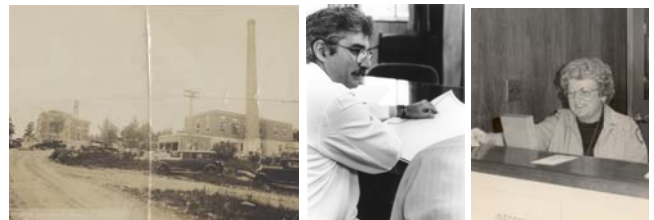
Left, the Hospital under construction in June 1932. Center, Dr. Sawicki in 1984. Right, Auxilian and volunteer Soni Cohn at the information desk.
